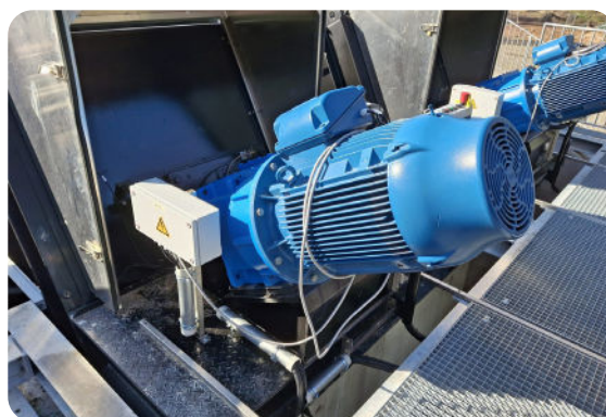
Drive unit of Landy semi-compact screw pump
