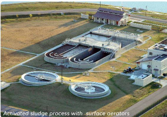
Activated sludge process with surface aerators
