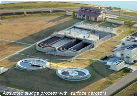
Activated sludge process with surface aerators
