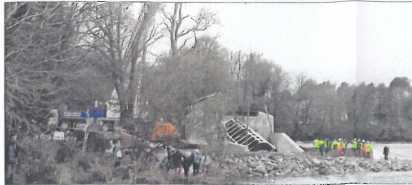
A crane lifts one of the two Archimedes screws into place
