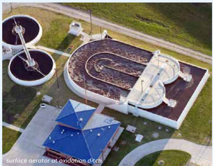
surface aerator at rectangular basin
